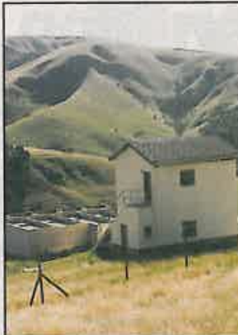
Nomponjwana community water-supply project
