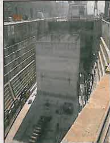
The gravity base structure
